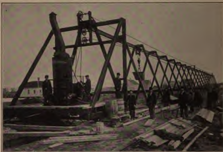
Trestle Cable Excavator Operating in Sewer Trench Construction. Figure 120.
